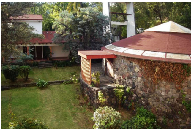
FIGURE 27 Exterior view of the chapel (2016)
